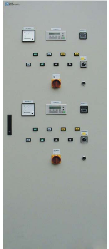
Control panel for 2 thruster motors
