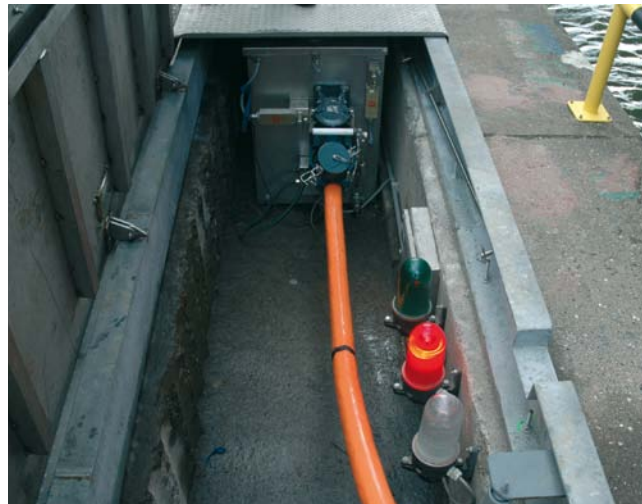
Socket station with connected HV-plug
