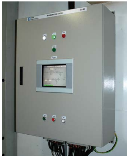
Ships management and control cabinet
